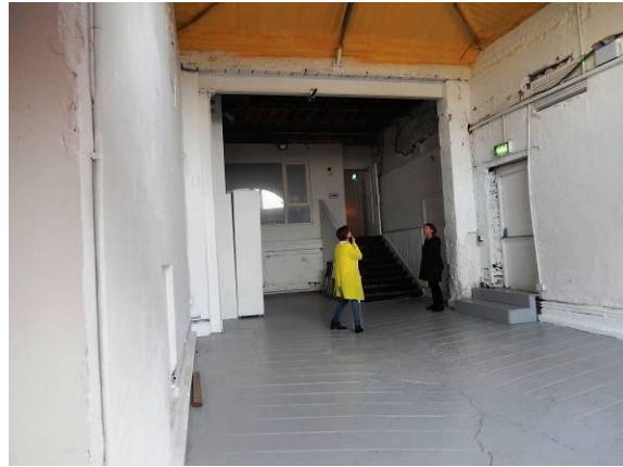
View E of ground floor of former fire station. The cross beam marks the beginning of the original house.
