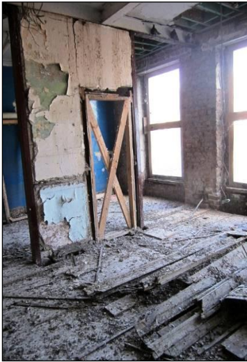
First floor removed walls.
