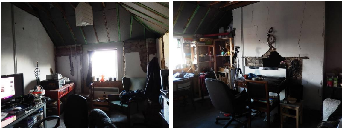
Views of second floor studios. Very little historic fabric survives at this level.
