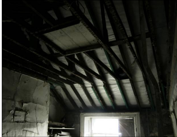
View of front room. Joinery stored to floor. Rear room with repaired roof timbers & new felt.
