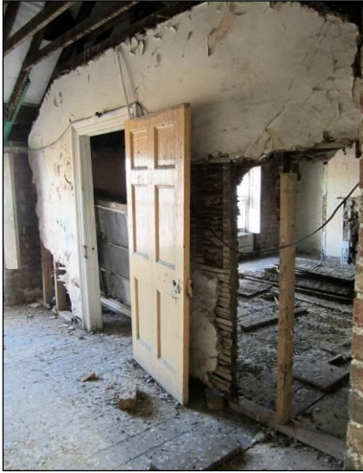
View of damaged wall to front room and rebuilt spine wall.
