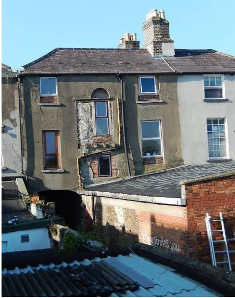
View of rear elevation of 190a
