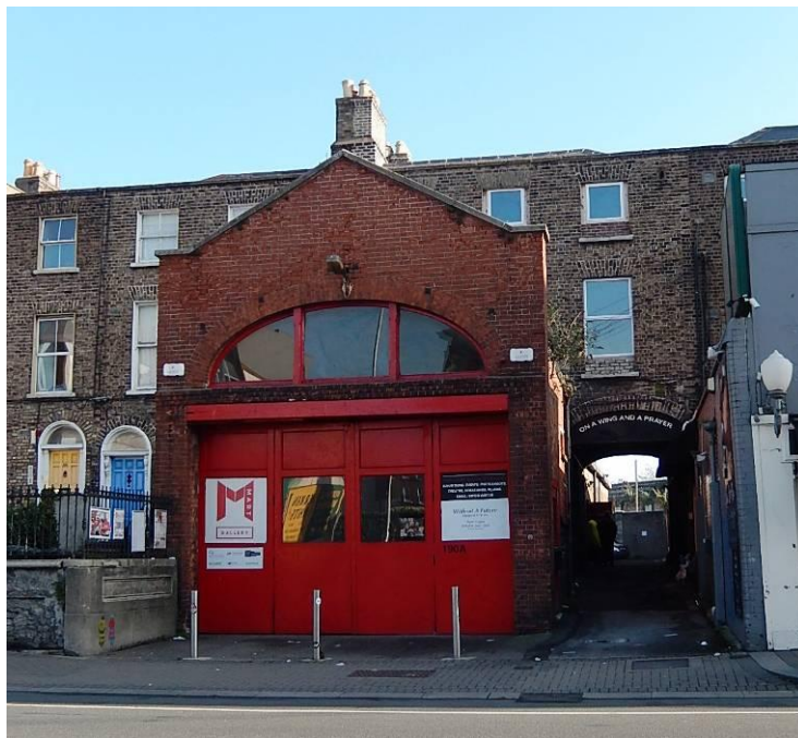
Photo of Structure
