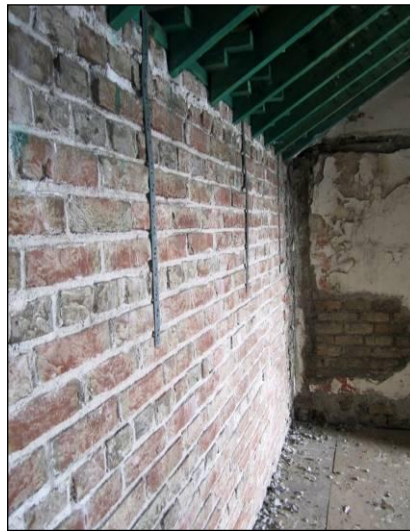
View of damaged wall to front room and rebuilt spine wall.
