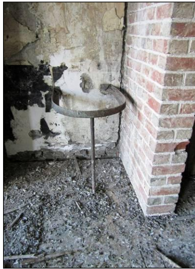
First floor location of security rail to firemen's pole.
