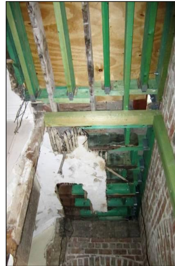
First floor ceiling, recent structural repairs.
